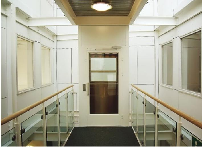
M6000 is a conventional lift built to EN81 standards and is ideal for installing within existing buildings where no shaft is apparent. Designed primarily for installation within, or alongside, a staircase the shaft can be supplied either fully or partially glazed, or even in a solid finish.
